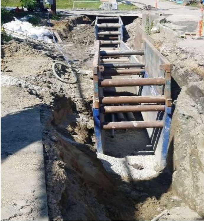
Fig 13: Pipe and duct bank install in College Brook cont. Viewing south. (7-15-19).
