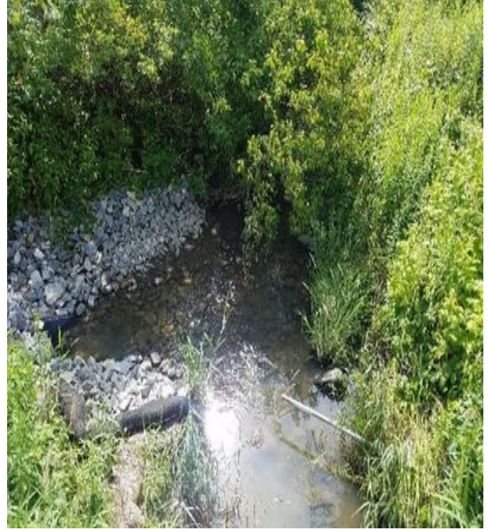
Fig 14: College Brook, downstream of trenching activities. Viewing west. (7-15-19).
