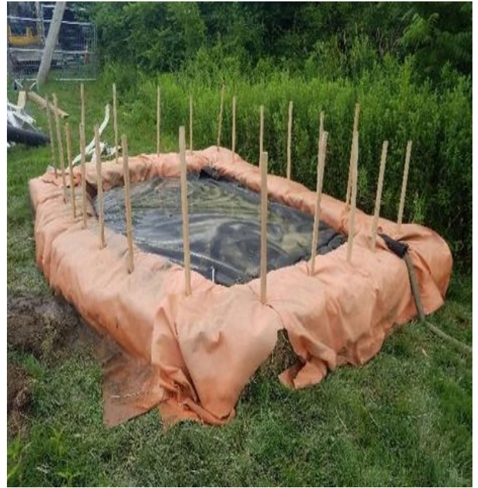
Fig 6: Newly built larger dewatering apparatus. Viewing north. (7-12-19).
