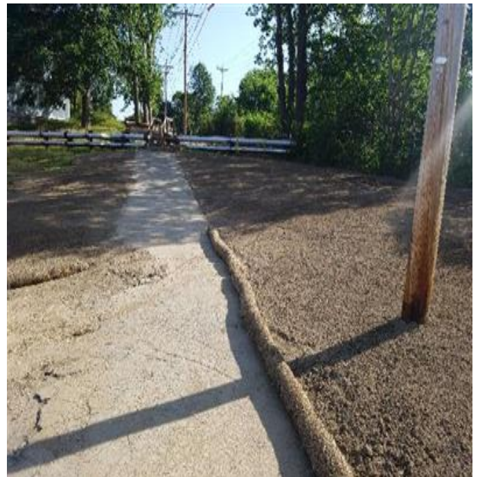
Fig 20: Restoration south of steam pipe, next to UNH field. Viewing north. (7-16-19).
