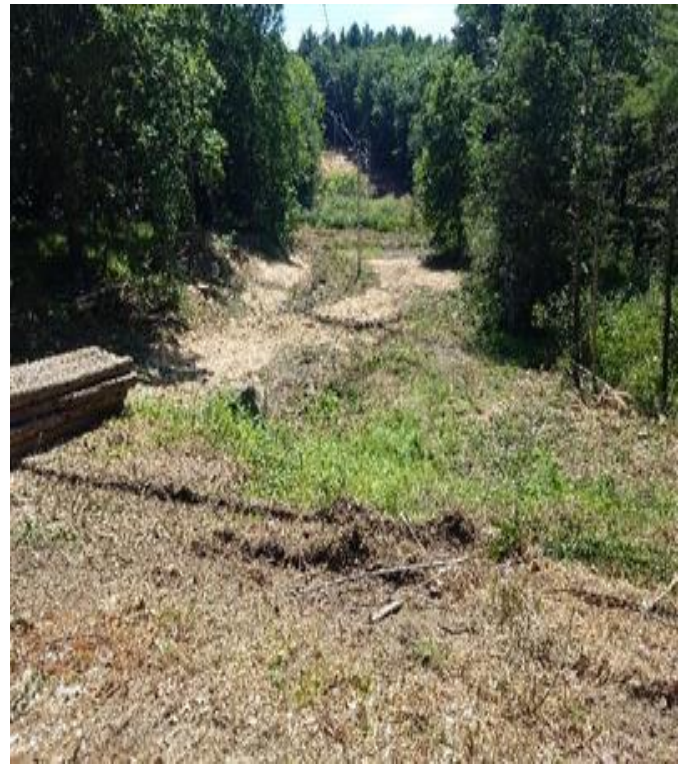
Fig 22: Clearing ROW towards Oyster River. Viewing south. (7-16-19).
