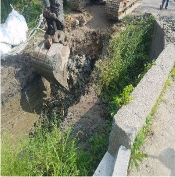
Fig 1: McCourt continues to excavate trench through College Brook. Viewing north. (7-11-19).
