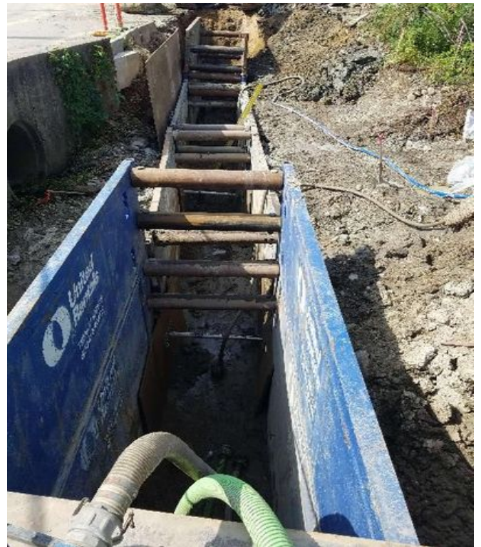
Fig 12: Pipe and duct bank install in College Brook. Viewing south. (7-15-19).
