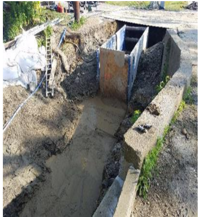
Fig 18: Float fill placed in trench running through College Brook. Viewing north. (7-16-19).
